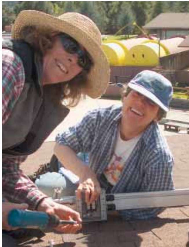
Kate Latham and Cecily Cahill mount a rooftop junction box.
