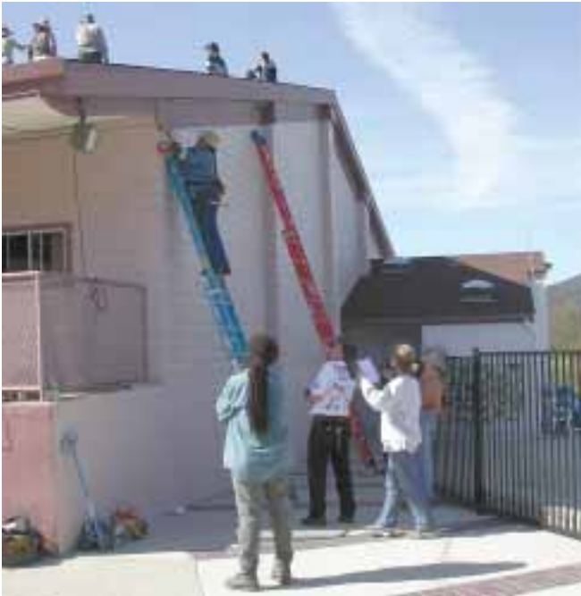
Installing the conduit run from the PVs to the inverter.
